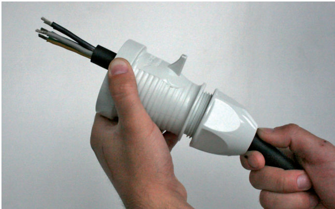
1. Dismantle approx. 50 mm of the cable and strip 10 mm of the wires, then feed the cable through the back part.
